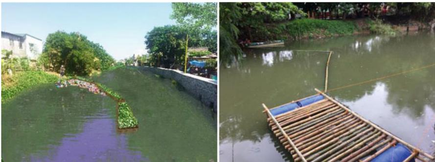
**Fig. 16** Innovative “Longganisa” to remove floating waste from rivers. 9b: The Longganisa constructed in November 2016 (in the back is the old way of collecting trash from the river with a boat)
